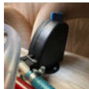
Frost Control drain valve
